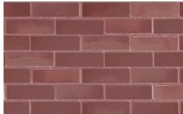
Brick Type 05 - New Cross Road frontage
